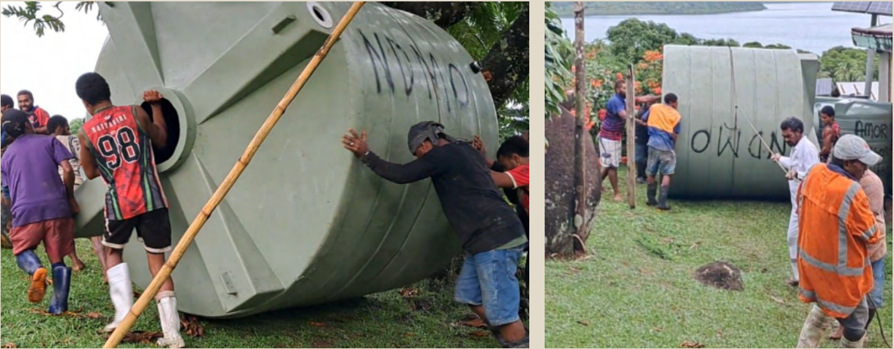
Pushing a 10,200 litre water tank up a 70-metre slope for its installation at Burelevu, Kadavu. Credit: Caritas Fiji.
