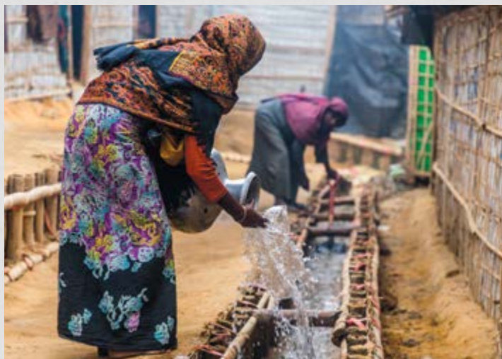
Through a Caritas cash-for-work activity, Rohingya refugees used local materials to build structures such as drainage and terraces to mitigate erosion and flooding in the refugee settlement. Photo: Christopher Reichert/CRS
